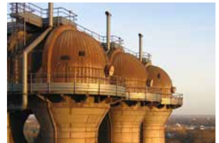
Blast furnace / stove dome
