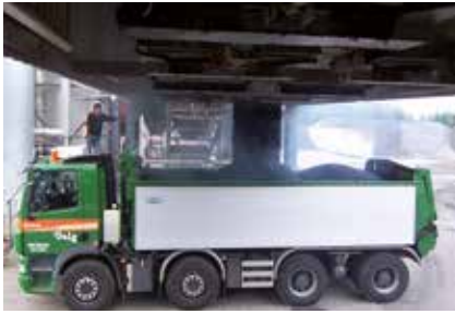
Asphalt and concrete mixing
