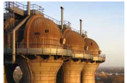
Blast furnace / stove dome
